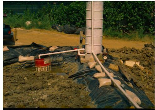
Bioreactor and Re-circulation system
